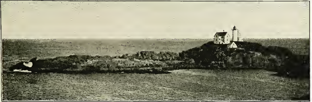
FIG. 67. — A lighthouse built on a small island at the tip of a cape.
